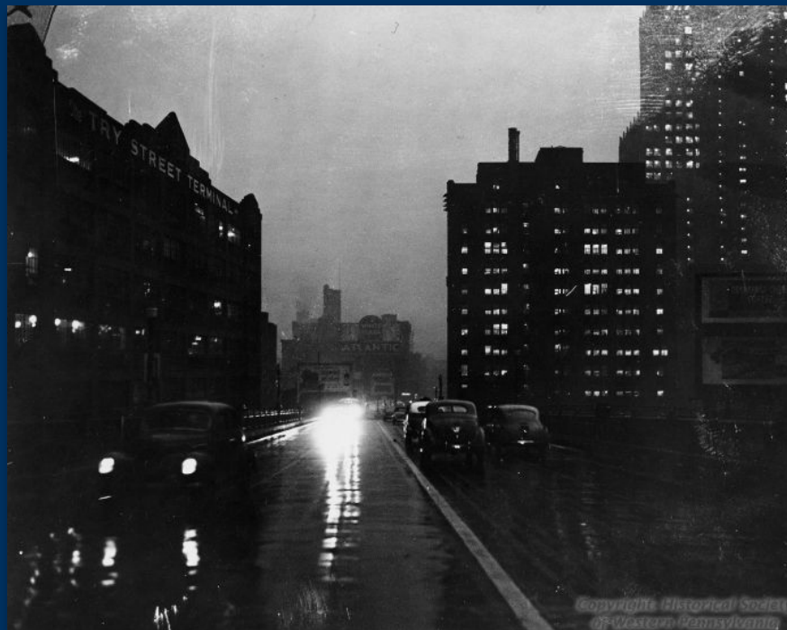
Before smoke control
